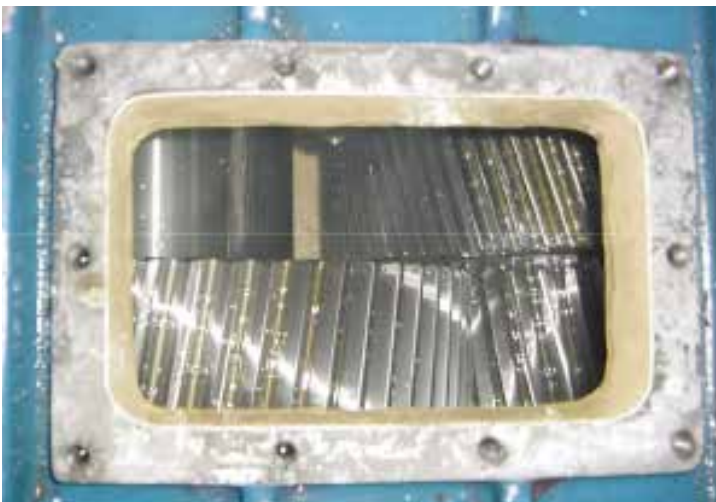
Figure 2 - Presence of foam in wind turbine gearbox
